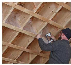
**Divide deep cavities.** Cavities deeper than 12 in. should be divided into cells using small pieces of netting spaced about 6 ft. o.c. The smaller space makes it easier to reach all corners, ensuring the cellulose is installed at the correct 3<sup>1</sup>/<sub>2</sub>-lb.- to 4-lb.-per-cu.-ft. density.
