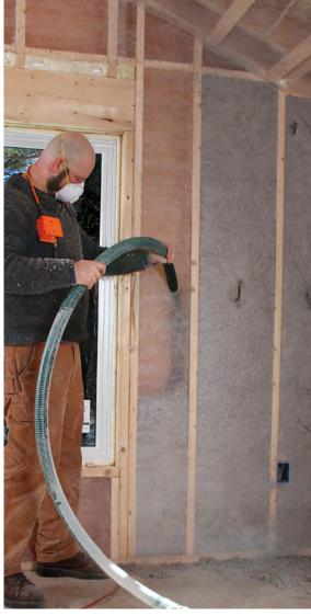
**Fill from the bottom up ...** In an 8-ft. or 9-ft. stud cavity, the whip is inserted near the middle and pushed all the way to the bottom plate. As the cavity fills, the whip is slowly withdrawn. When the cavity is half filled, the whip is removed.
