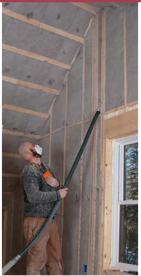
**Beware of blind spots.** Odd-shaped and hidden cavities are marked with a Sharpie during the netting stage so the insulator remembers to fill these spaces. Blind corners created by adjoining walls are best filled through multiple holes spaced a couple of feet apart, with the hose plunged horizontally into the hidden part of the cavity. Cavities smaller than 2 in. are filled with canned spray foam.
