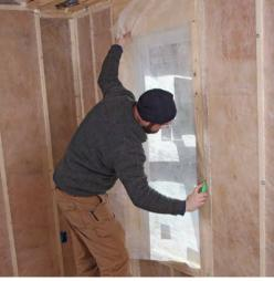
**Trim around doors and windows.** Excess netting is trimmed along the bottom plate and around the perimeter of framed openings where it covers doors and windows. The nonwoven material cuts easily with a fresh blade.
