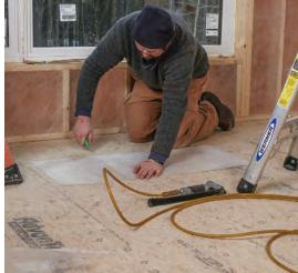
**Cut small pieces on the floor.** Precision isn't critical for the small pieces of netting used to divide cavities, but using a measured piece as a template helps speed the work of cutting a stack of the small rectangles needed to divide the 16-in.-deep rafter cavities.
