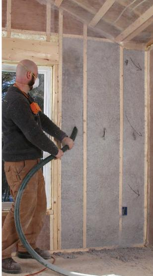
... and then from the top down. With the reinserted whip pushed to the top plate, the cavity is then filled from the top down. As the cavity fills, the whip is backed out and withdrawn. Installed correctly, the cellulose is packed tight enough that patching the hole is unnecessary.
