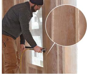
**Lip-stitch the studs.** Once the netting is facestapled around the assembly perimeter, it's stapled to both front corners of the studs or framing members with staples placed about 1 in. apart. This method, called lip-stitching, draws the netting even tighter across the cavity to help prevent bulging.
