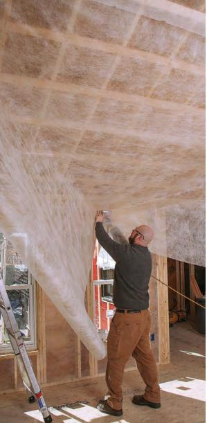
**Drape and pull.** Ceiling cavities are tackled much the same as walls. The netting is fastened to the ridge and allowed to hang down, then pulled tight and fastened along the bottoms of the rafters before lip-stitching.
